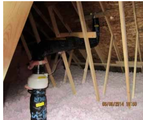
Figure 4. Example of Insulated Pipe
