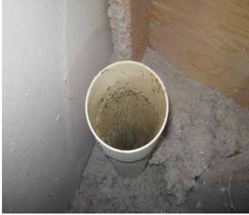
Figure 5. Example of Pipe Venting Into Attic
